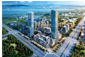
Walsin Centro Nanjing, China
